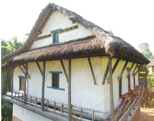
Figure 8: Use of tundals and wooden posts
