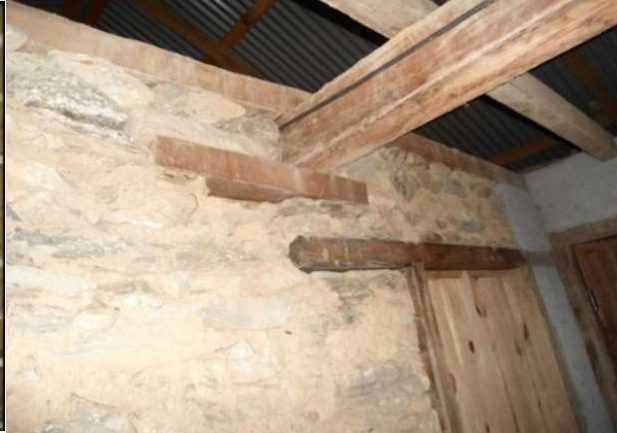
Figure 6: Use of Wedges to make the Wall Tight
