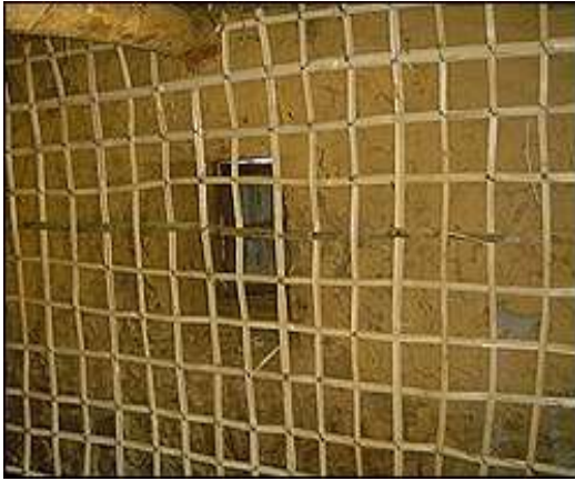
Figure 7: Bamboo reinforcement for retrofitting
